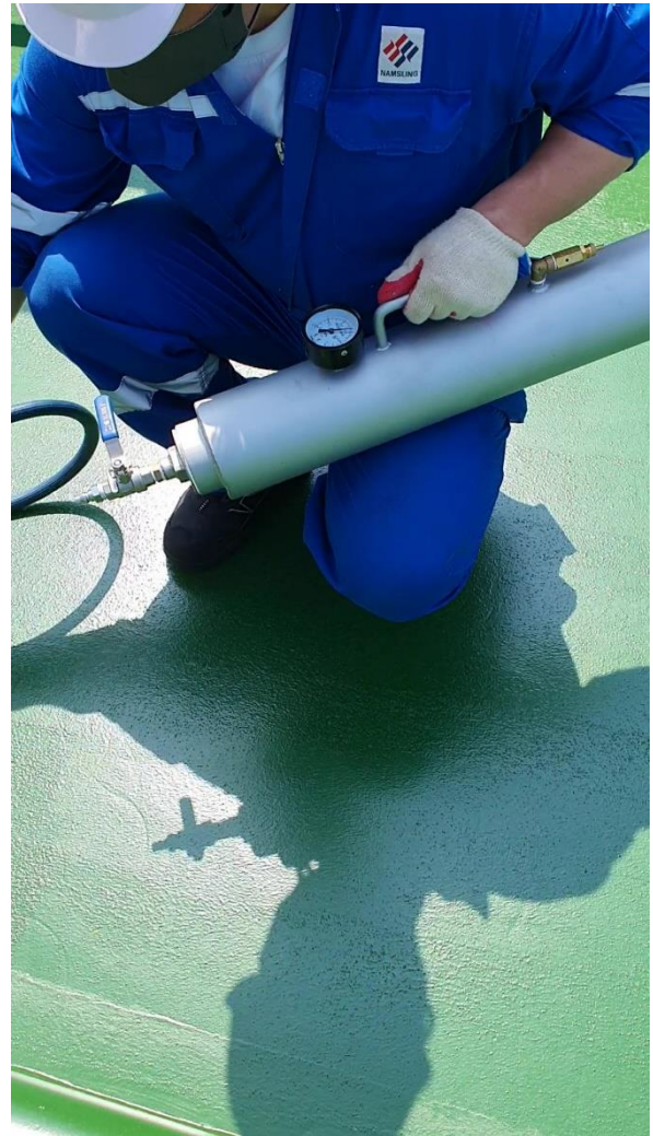
Check the closed valve and disconnect the air hose.
