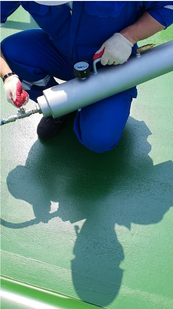
When air is supplied to the desired pressure, close the valve.
